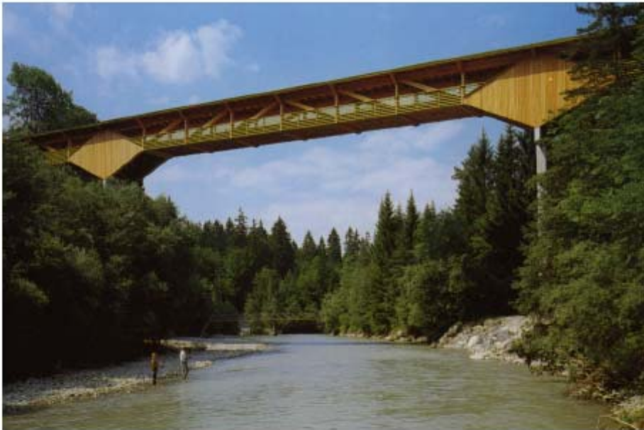
Bridge across river Sinne (Switzerland)
