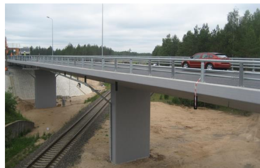
Fig. 3. Cross section and elevation of bridge on road A12 over Railway Rīga - Rēzekne. FE model constructed as a plate-strut 3D
