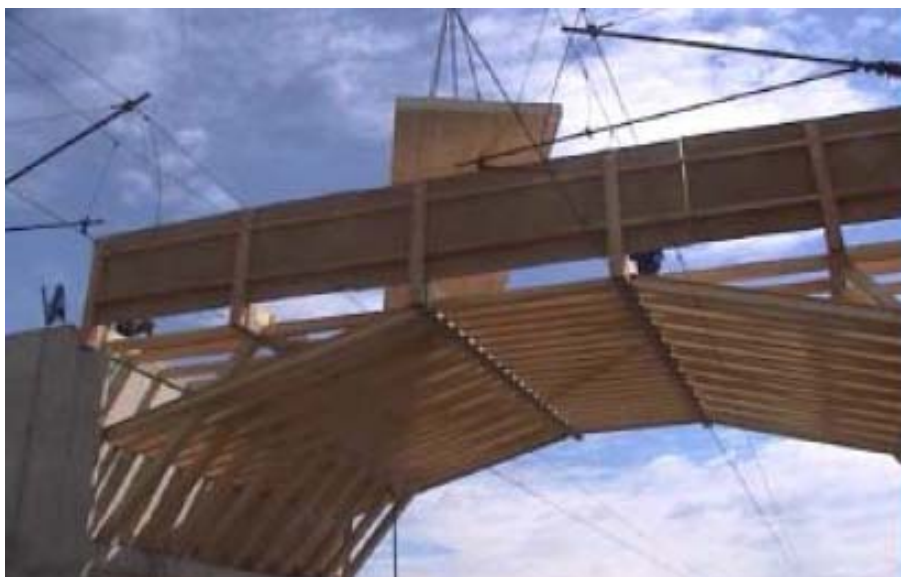
Pedestrian bridges with the decking made of CLT (Feldbach, Austria)
