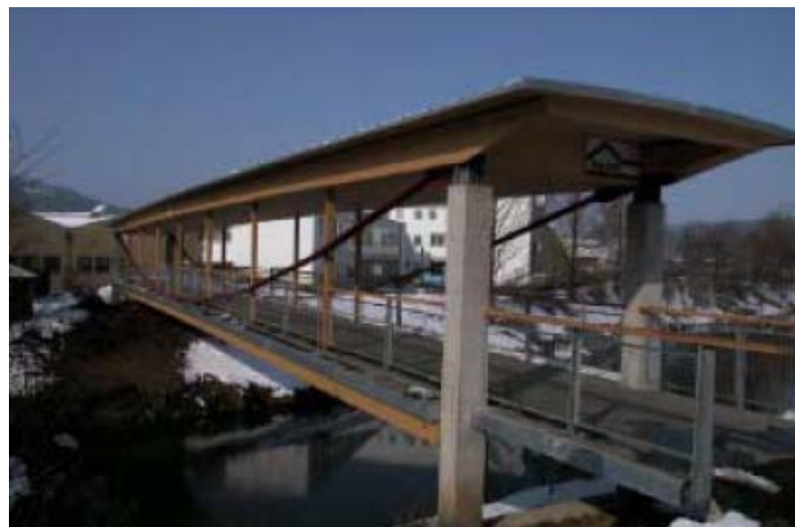
Pedestrian bridges with the decking made of CLT (Feldbach, Austria)
