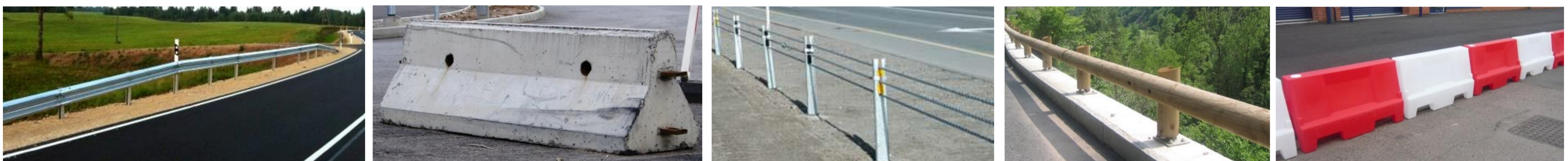
Fig. 8-12. Different type of road barriers.
