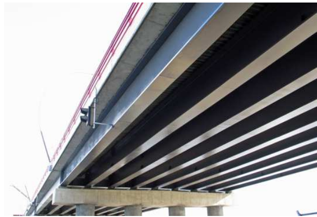
Figure 6: Bridge over Venta River
