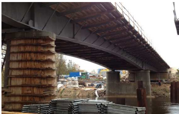
Figure 9: Bridge over Gauja River
